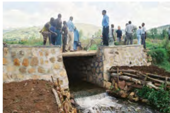
A rehabilitated bridge in Gituza commune © Francis Dobbs, World Bank.
